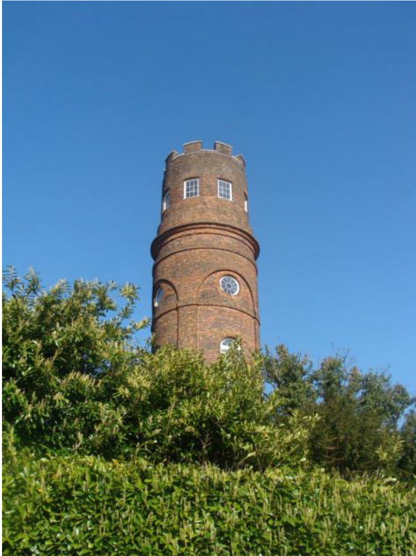
Picture 5. The remarkable late 18th century tower for J. Stratton which dominates the local scene.
