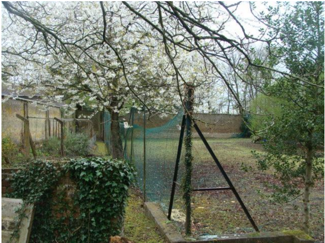
Picture 25 and 26. Part of wall range to east of Little Berkhamsted House worthy of retention.
